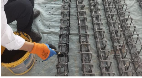
Fig. 3.3 Anti-corrosion paint is applied
