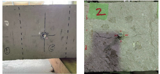
(a) 拡底 60 No.2 (割裂破壊) (b) 拡張 60 No.2 (割裂破壊)
