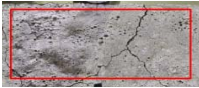
Cracking caused by ASR
