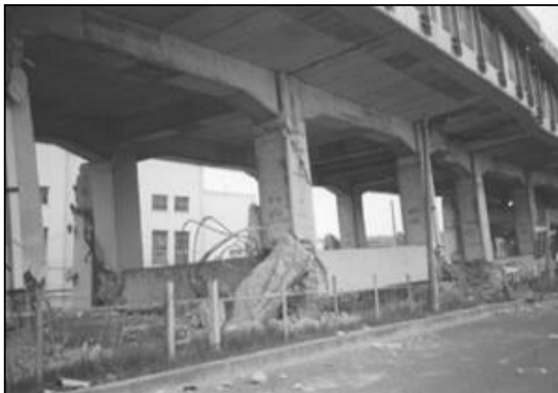
Figure 5.7 Damaged conditions of Hansui R5 (Miki.2004)
