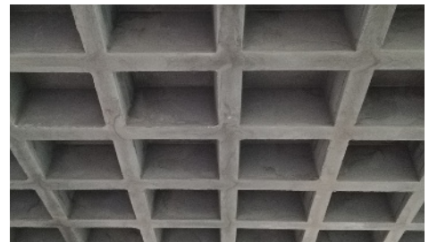
(c)UFC (硬化後：UFC 床版の下面)
