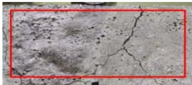
Cracking caused by ASR
