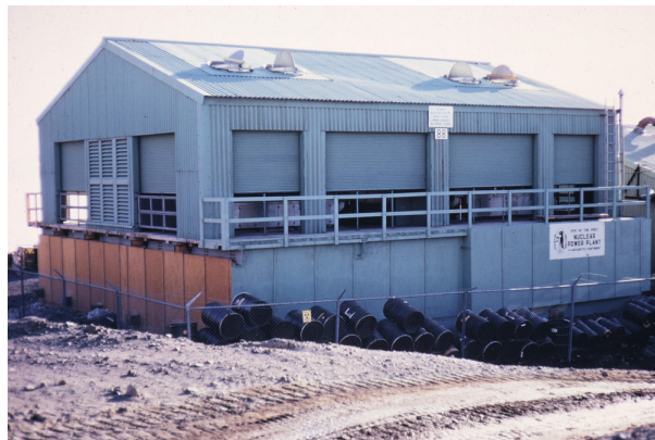
Exterior view of McMurdo Station nuclear power plant with drums stacked along the wall. Date 1967-68 season Antarctica New Zealand Collection https://adam.antarcticnz.govt.nz/nodes/view/6083
