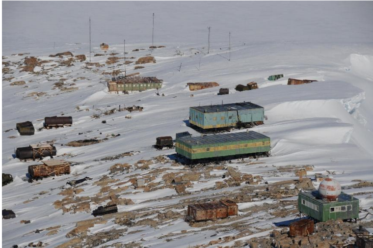
Aerial inspection of Leningradskaya Station (Russian Federation) in East Antarctica, conducted by Australia in January 2011. Leningradskaya was open in 1971 and closed as a permanent year-round station in 1991. The station is currently referred to as “mothballed”. Copyright Australian Antarctic Division
